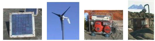
We really rough it here, what with the microwave, bread maker, stereo, gas stove, gas heaters, computers, phone, email etc., but all this needs power. We try to run from 12V batteries for most of the time, and keep these charged from a combination of solar and wind power. There are a few things that need 240v, and there are times when there is no wind and very little sun, so we have a 5kW generator to fill in.
